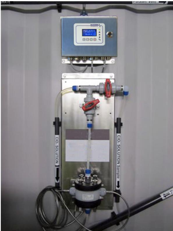
*Kemtrak DCP007 Prozessphotometer CIO<sub>2</sub> Installation*
